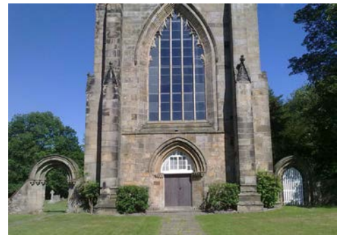
Ongoing repairs and maintenance at Beauchief Abbey
