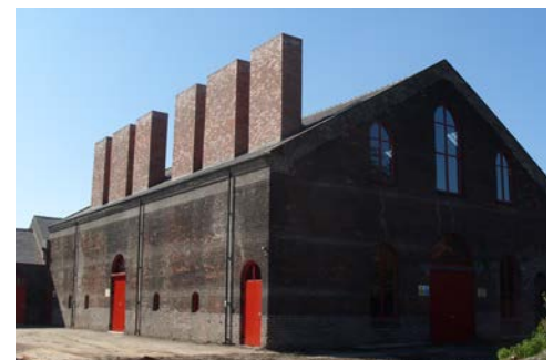
Envelope Repairs to the Crucible Workshops, Darnall
