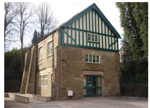
Residential Conversion of Annexe Buildings for Kingfield Centre for Sheffield Jewish Congregation
