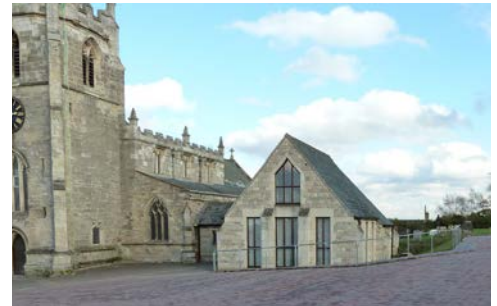
New parking and disabled access provisions at St. James' Church, South Anston
