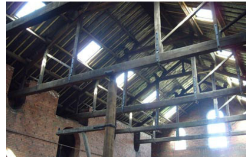
Envelope Repairs to the Crucible Workshops, Darnall
