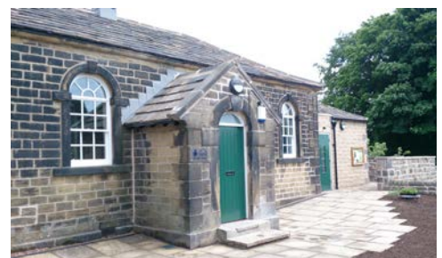
Alterations, Repairs and Extension to the Former Endowed Reading Room, Grenoside
